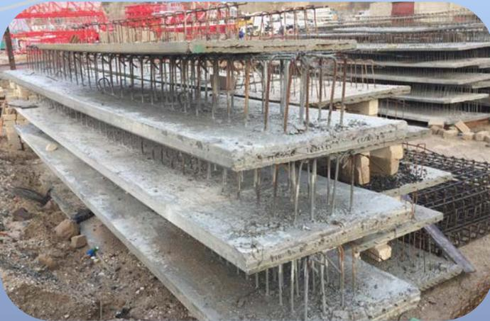
The manufacturing system of prestressed preloses TECNOSPAN, provides a production structure which facilitates the execution of the works. This system was born in order to cover the needs of the markets where the buildings requires large open spaces without needing to provide large tonnage machinery for its installation.
